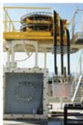
Figure 8—Hoses reel storage system and the connection head maintenance & storage platform
